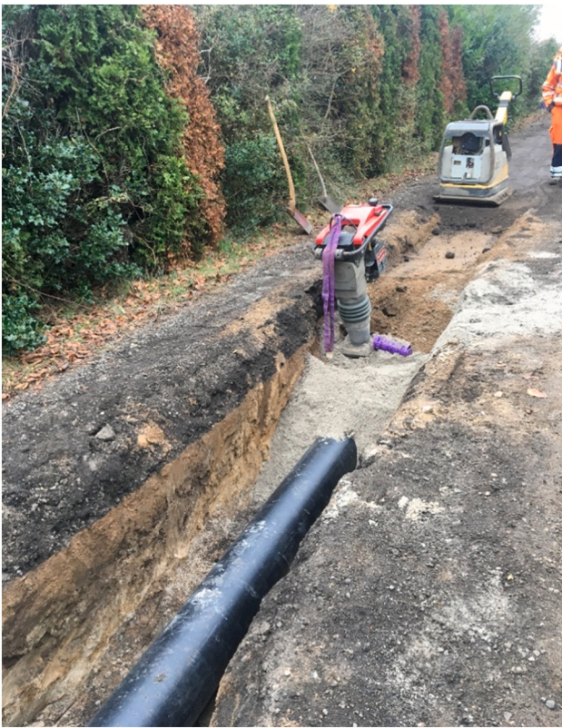
Image 2. District heating pipes for a new housing area in Odense are buried underground on a street that has been closed during the digging work. Image by the author.
