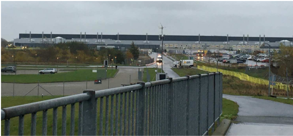
Image 1. The Meta datacenter in Odense, Denmark, in November 2020.
